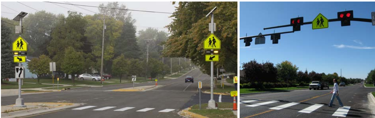
Rectangular rapid-flash beacon (left) and high-intensity activated crosswalk beacon (right).
