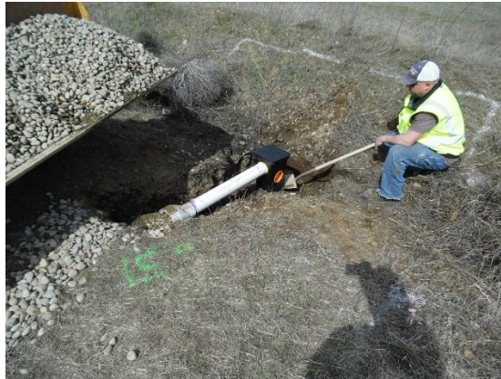
Step 2, make and install outfall equipment
