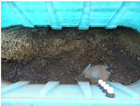
Let all tanks drain and evaporate for two weeks
