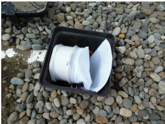
Step 5, install socks in all 8 outfall catchments
