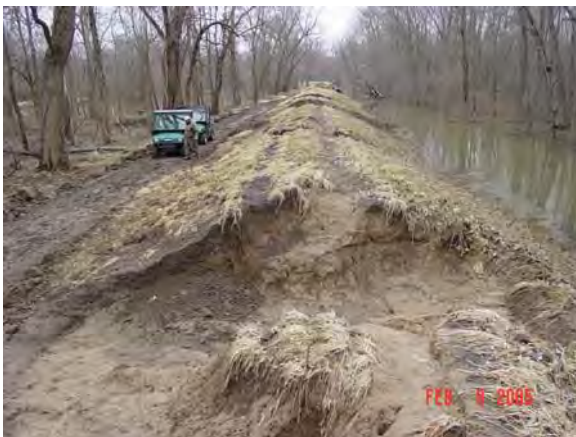
Figure 6.2 and 6.3, Levee breaches along the Wabash River
