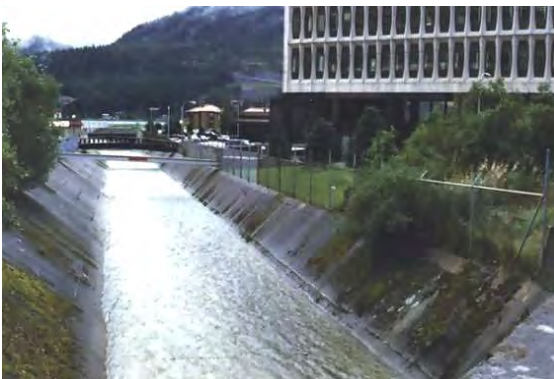
Figure 2.74 ACCEPTABLE concrete lined channel. (AK)
