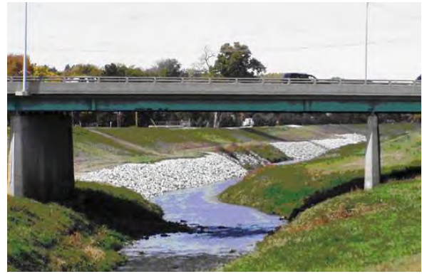
Figure 2.26 ACCEPTABLE riprap for erosion control. (NE)
