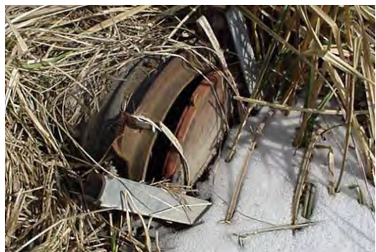
Figure 2.66 UNACCEPTABLE flap gate in earthen levee. (Broken hinge and vegetation)
