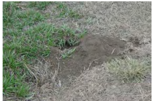
Figure 2.20 Animal burrow in a levee. (IA)
