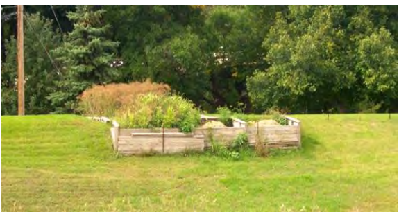
Figure 2.13 UNACCEPTABLE encroachment. Gardens and compost bins located on levee crest and riverward slope. (ND)
