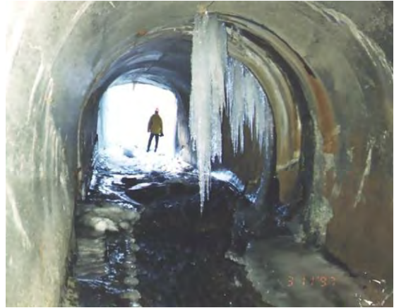
Figure 2.58 Concrete drainage tunnel. (AK)
