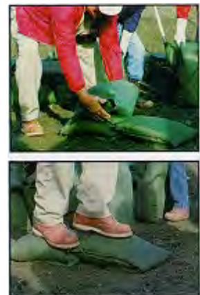
Place each succeeding bag tightly against and partially overlapping the previous one. Compact and shape each bag by walking on it.
