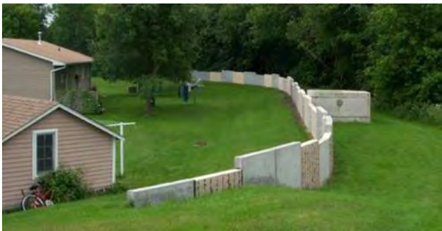
Figure 2.50 ACCEPTABLE. decorative floodwall is in straight alignment, with no tilting or spalling, and all joints are tight together. (MN)
