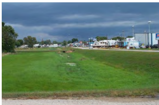
Figure 2.54 ACCEPTABLE interior drainage channel. (IA)
