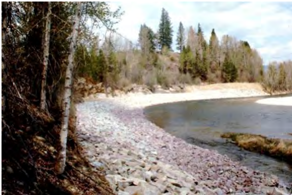
Figure 2.25 ACCEPTABLE riprap for erosion control. (MT)
