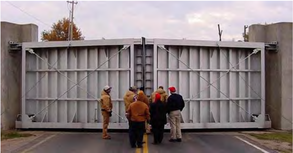
Figure 2.42 ACCEPTABLE floodgate in a levee. (KS)
