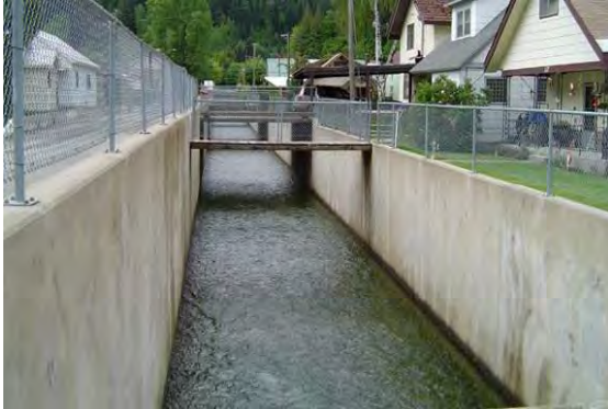
Figure 2.72 ACCEPTABLE concrete lined flood control channel. (ID)
