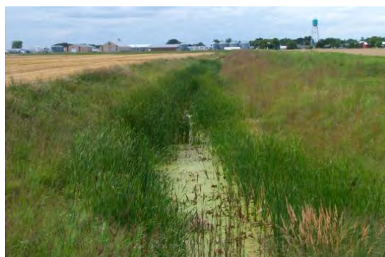
Figure 2.55 MINIMALLY ACCEPTABLE vegetation (cat tails and bull rushes) in interior drainage ditch. (MN)
