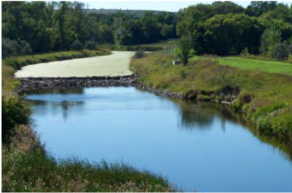
Figure 2.15 UNACCEPTABLE. Slope failure and erosion caused by inadequate channel bottom and side slope protection. This was a direct result of bottom scouring that undercut the levee slope and erosion caused by turbulent flow at the end of the bank protection. (ND)
