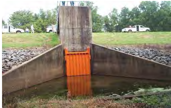
Figure 2.63 ACCEPTABLE culvert gate. (LA)
