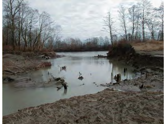
Figure 6.1, Levee breach in Lynden, WA
