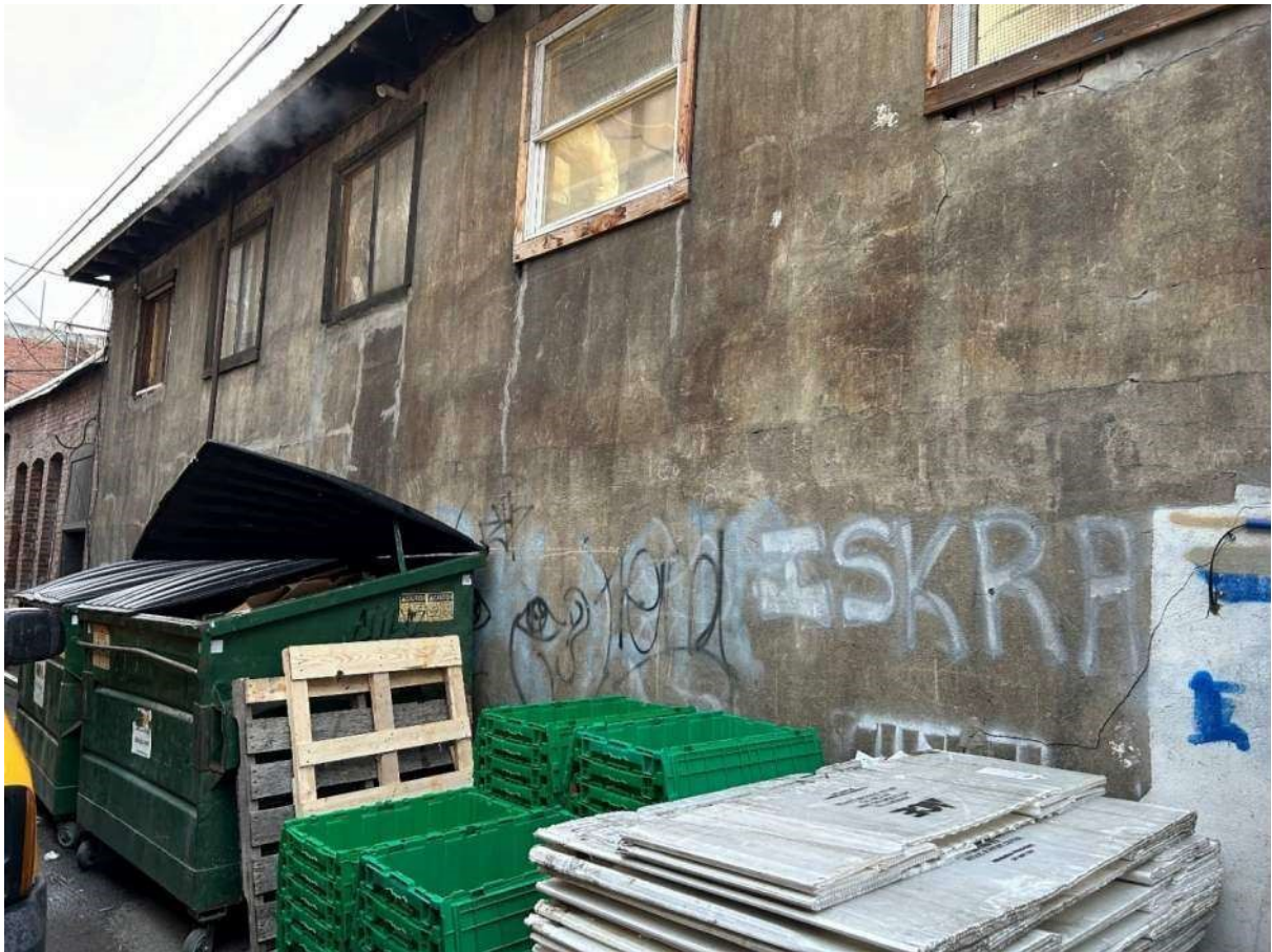
Looking southeast at the gray stucco siding of the warehouse addition. Some exposed terra cotta block is visible under the window on the right side of the photo.
