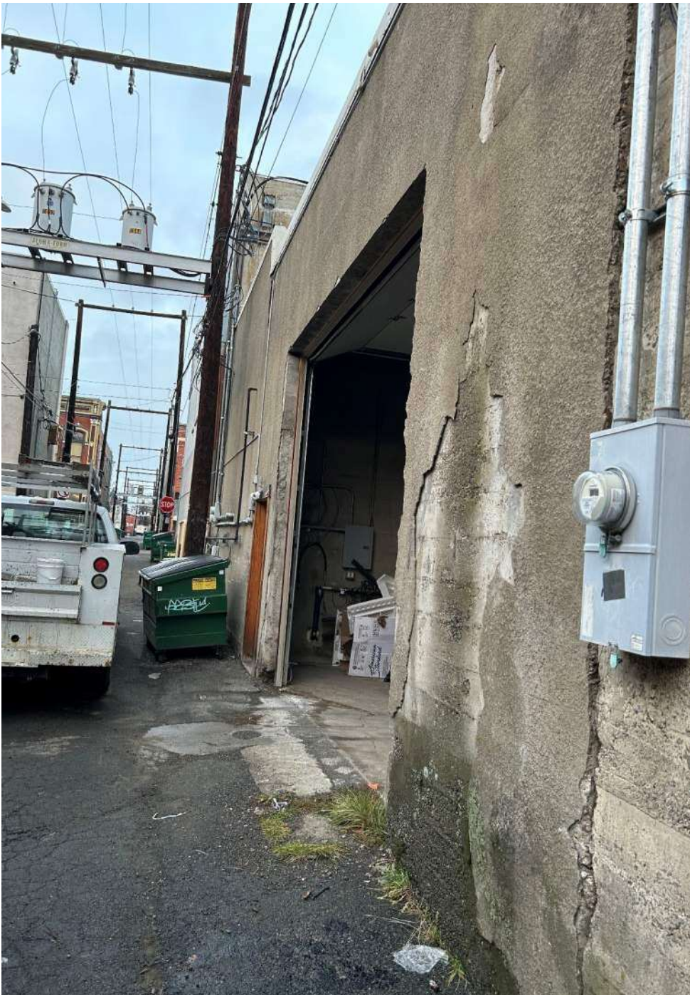
Across the alley on the north side is a warehouse building occupied by Paramount Electric for storage.
