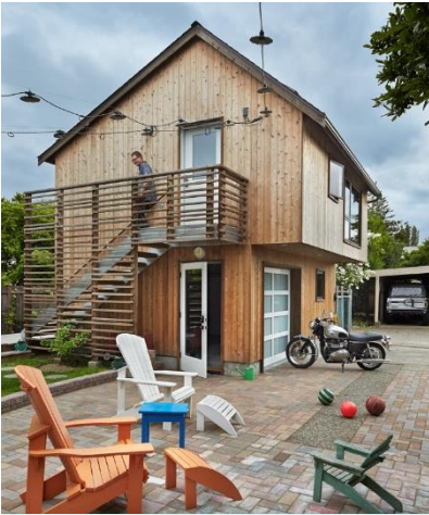
Detached accessory dwelling unit (photo SHKS Architects)
