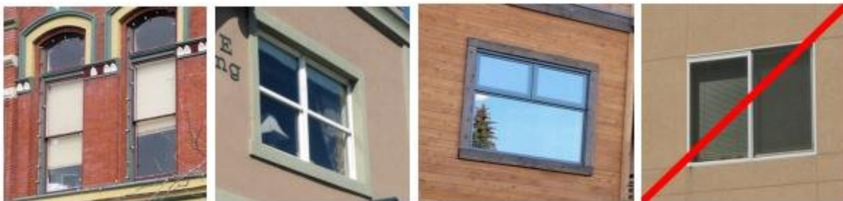
Figure 15.530.040(E). Acceptable and unacceptable (far right image) window design on upper floors. Note that the windows in the brick building on the left are recessed from the facade. The windows in the middle images include trim. The image on the right includes no trim or recess/projection, and thus would not be permitted.
