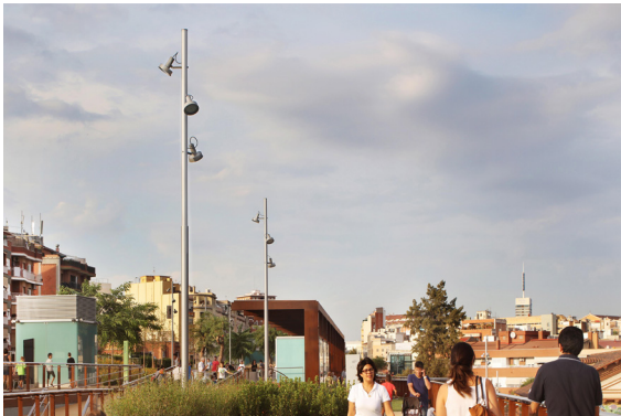
lighting: lights and event poles
