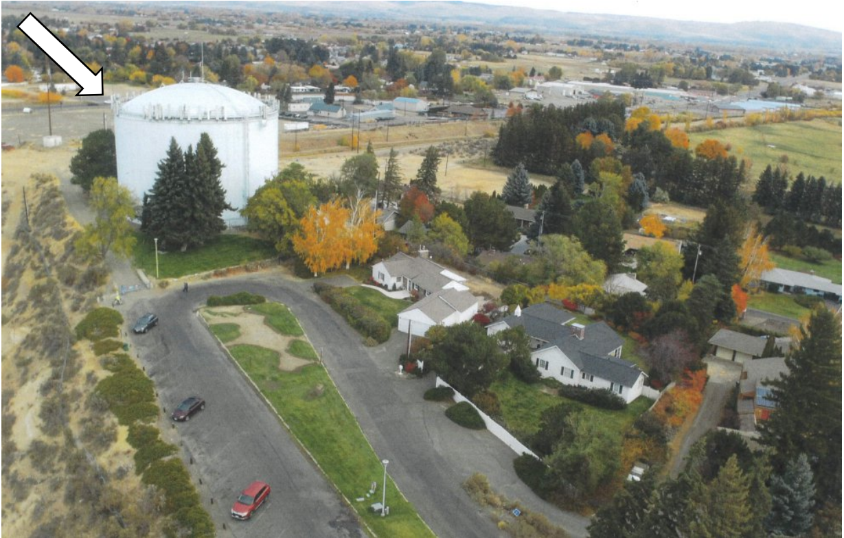
Craig's Hill Reservoir - view from the south (above)
