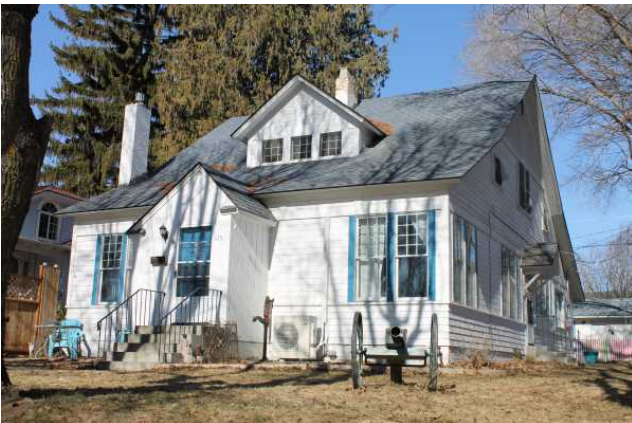
south and east facades
