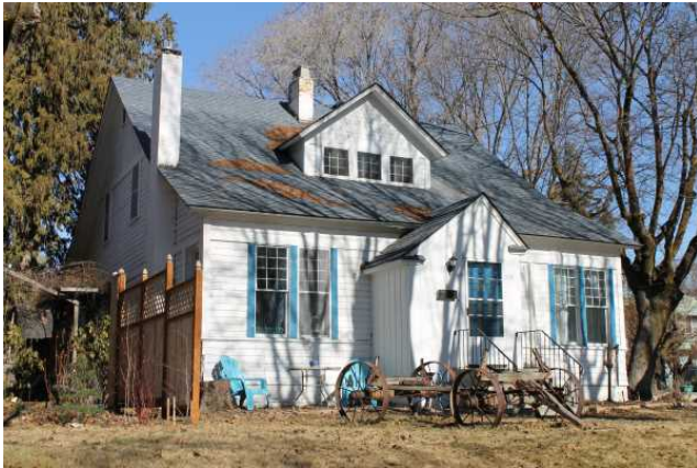
south and west facades
