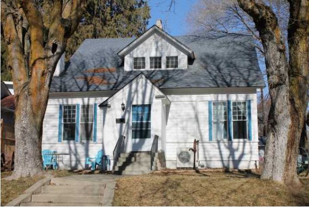
primary (south) facade
