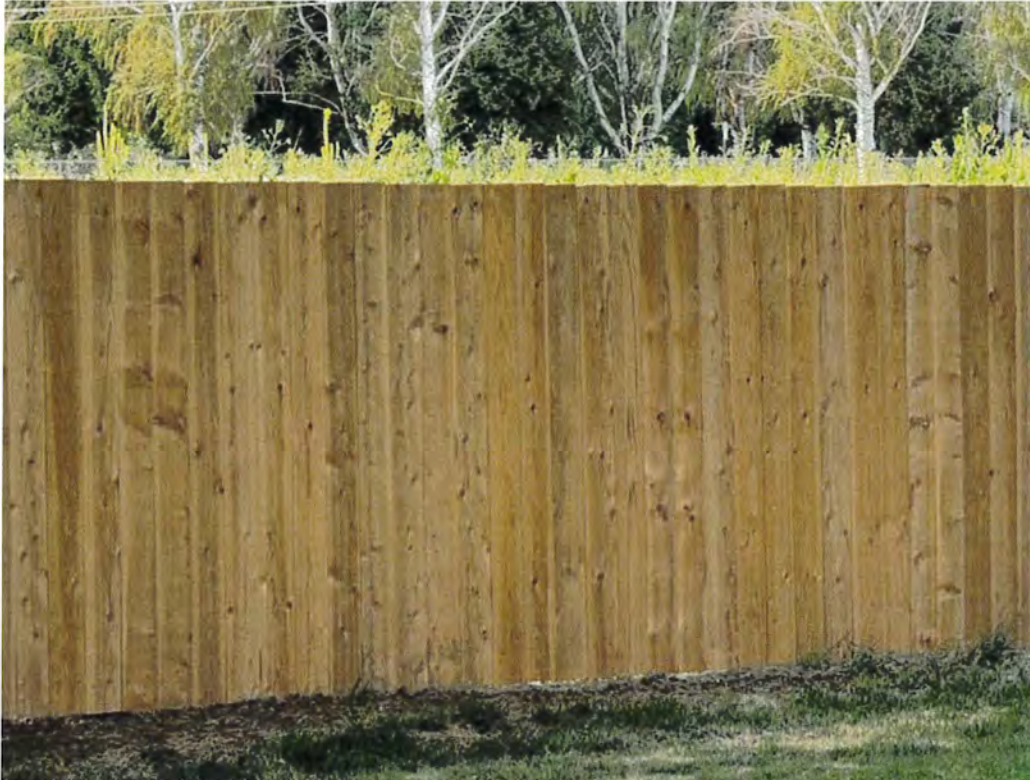
Six foot cedar fence, weeds are above fence
