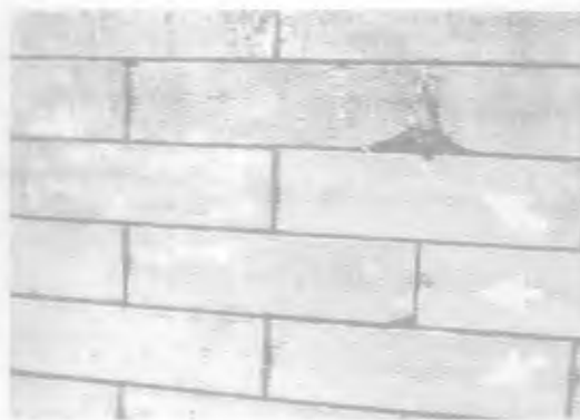
Figure 11. Rinsing with high-pressure water following chemical cleaning has left a horizontal line of abrasion across the bricks on this late-19th century row house.
