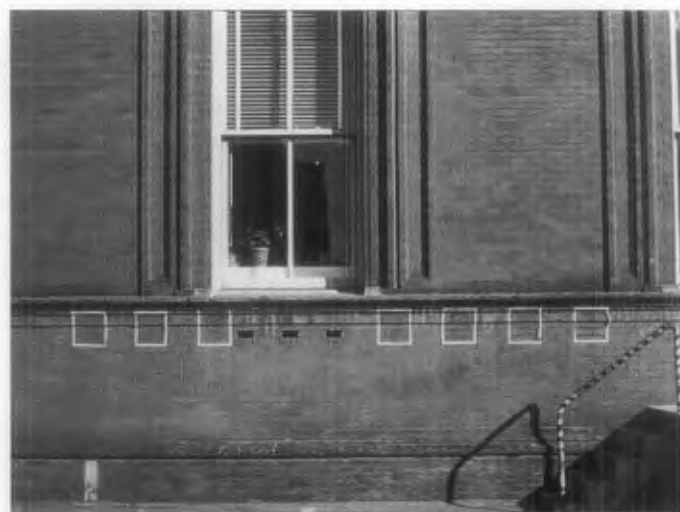
Figure 22. Cleaning test areas may be quite small at first and gradually increase in size as testing determines the "gentlest means possible". Photo: Frances Gale.
