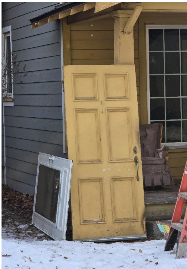
Existing/ Original Door:
