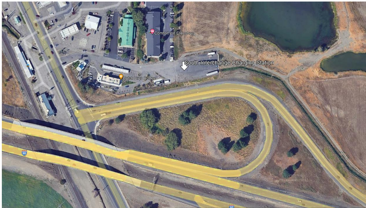
FIGURE 23: EV CHARGING STATION, SOUTH I-90 INTERCHANGE SITE
