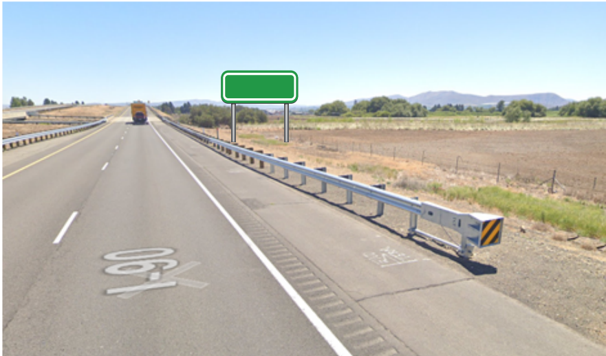
Eastbound I-90, approx. Milepost 109.06 New full-size sign
