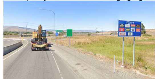
EB ramp: May need to revise existing signage.
