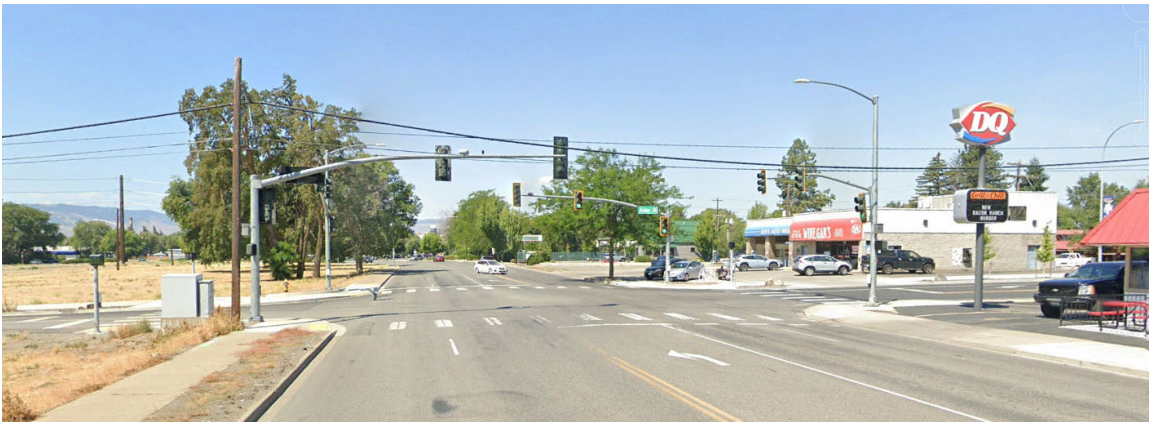
University Way Looking West at Alder Street Note: Location of a KSI
