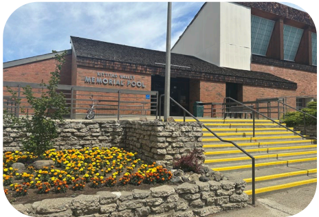
Replace/renovate Kittitas Valley Memorial Pool
