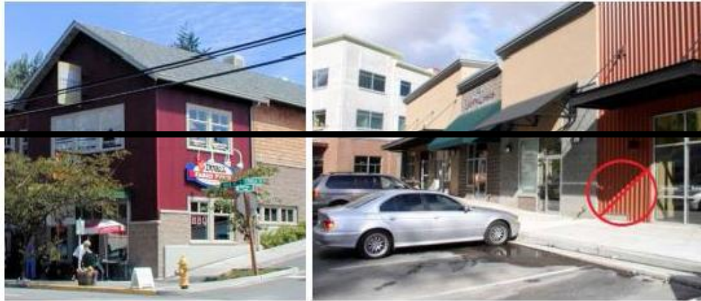
Figure 15.530.050(C). Acceptable and unacceptable metal siding examples. Notice the corner and window trim and use of concrete block near the ground level on the left image. The circled area on the right includes metal siding all the way to the ground, which is prohibited.
