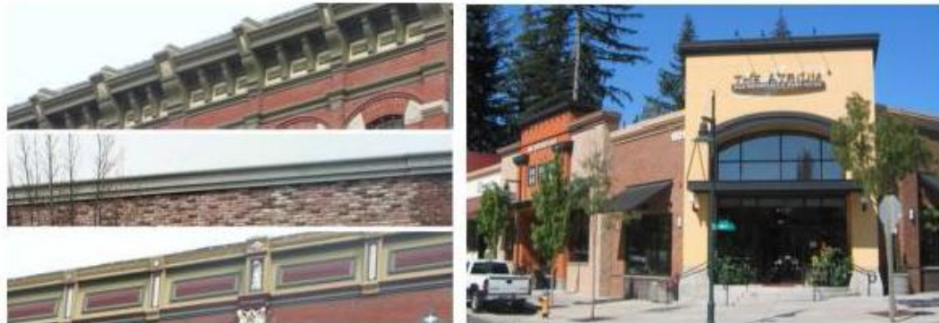
Figure 15.530.030(E)(1). Decorative cornice examples on existing historic buildings downtown (left images). The right image shows examples of a variety of cornice designs on a new building.
