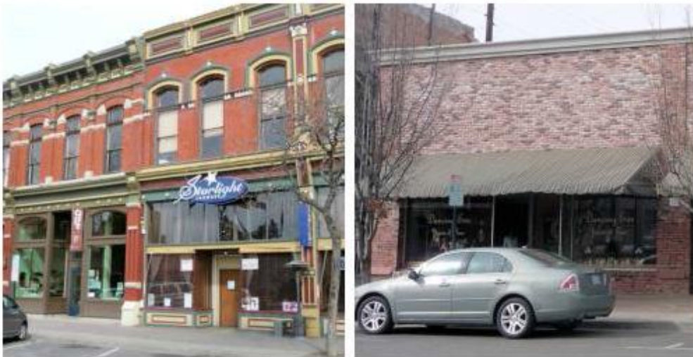
Figure 15.510.050(C). Current storefront examples. Note the large storefront windows and recessed entries in the left image. In the right image, note the relatively tall height of the single-story building. The height helps to add a sense of enclosure to the street.
