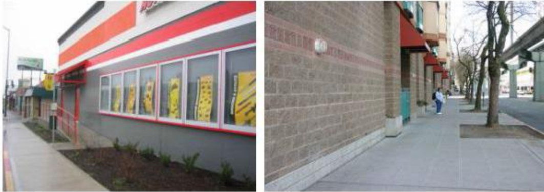
Figure 15.510.050(D). These facades do not meet the storefront standards. The tack-on display cases in the left image do not qualify as transparent window area.
