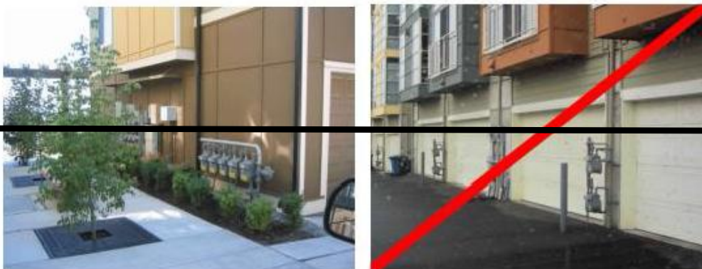
Figure 15.520.060(C). Good and bad utility meter configurations. The examples on the left are consolidated and somewhat screened by landscaping elements, whereas the right examples are exposed and degrade the character of these townhouses.
