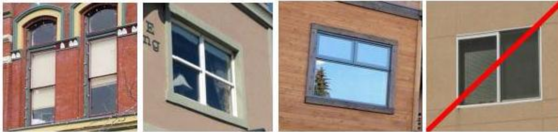
Figure 15.530.040(E). Acceptable and unacceptable Compliant and non-compliant (far right image) window design on upper floors. Note that the windows in the brick building on the left are recessed from the facade. The windows in the middle images include trim; the un-recessed window is trimmed with color contrasting from base building color . The image on the right includes no trim or recess/projection, and thus would not be permitted.
