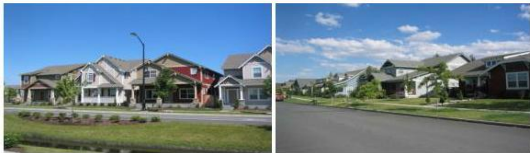
Figure 15.420.030(E)(1). The above dwellings feature a good diversity of yard spaces , facade designs, colors and rooflines.
