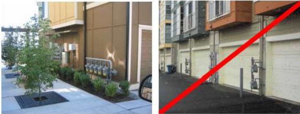
Figure 15.530.045(A). Compliant and non-compliant utility meter screening. The examples on the left are screened by landscaping elements; the right examples are exposed.
