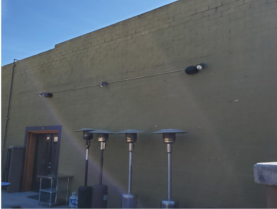
412 N. Main St – North Façade
