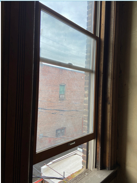
Example of existing retrofit windows with wood sashes in vinyl tracks.
