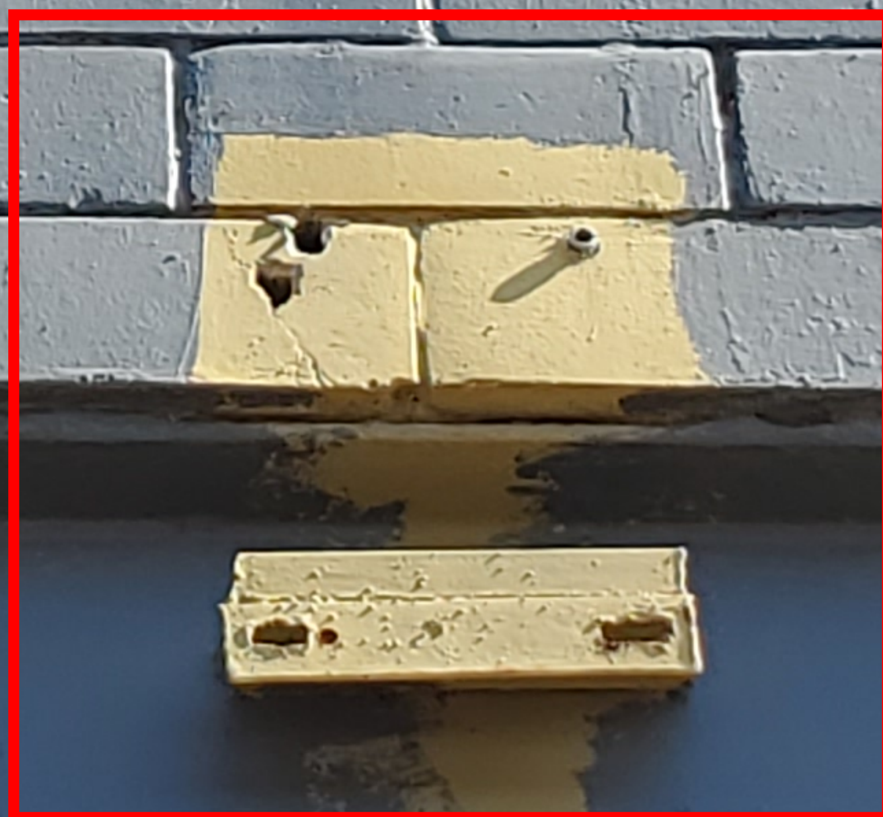
Existing Mount for Sign
