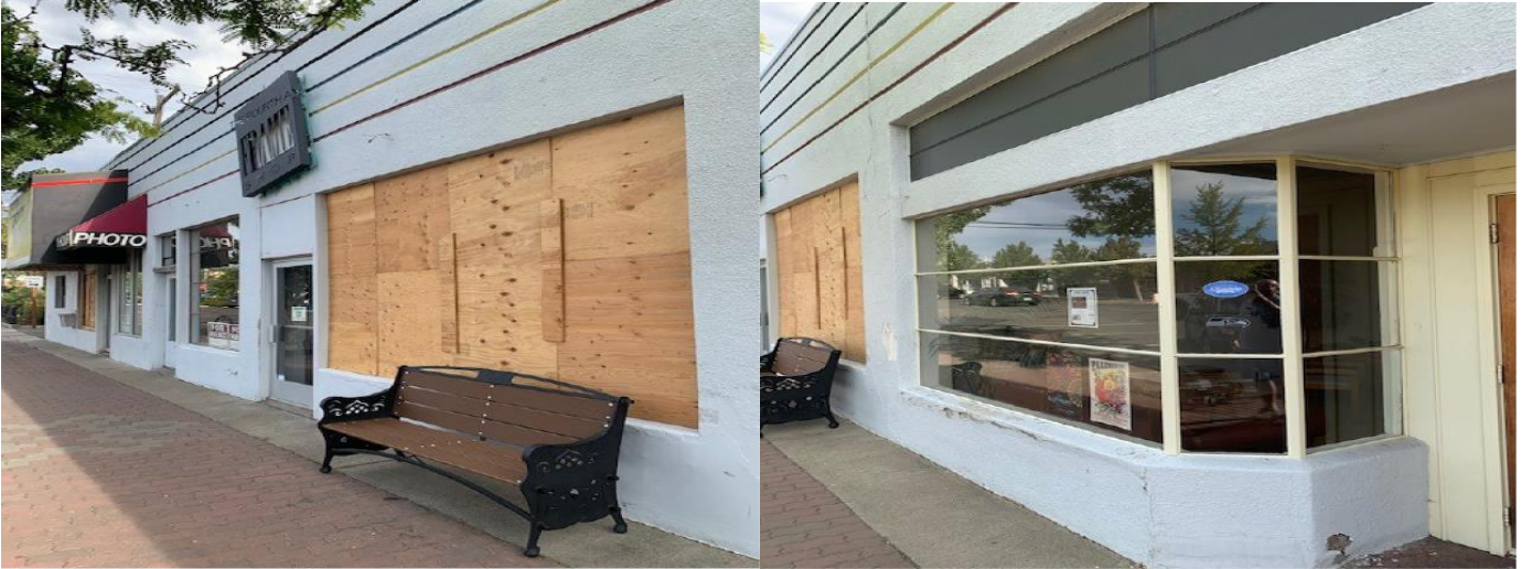
McCORMACK BUILDING WINDOWS BEFORE
