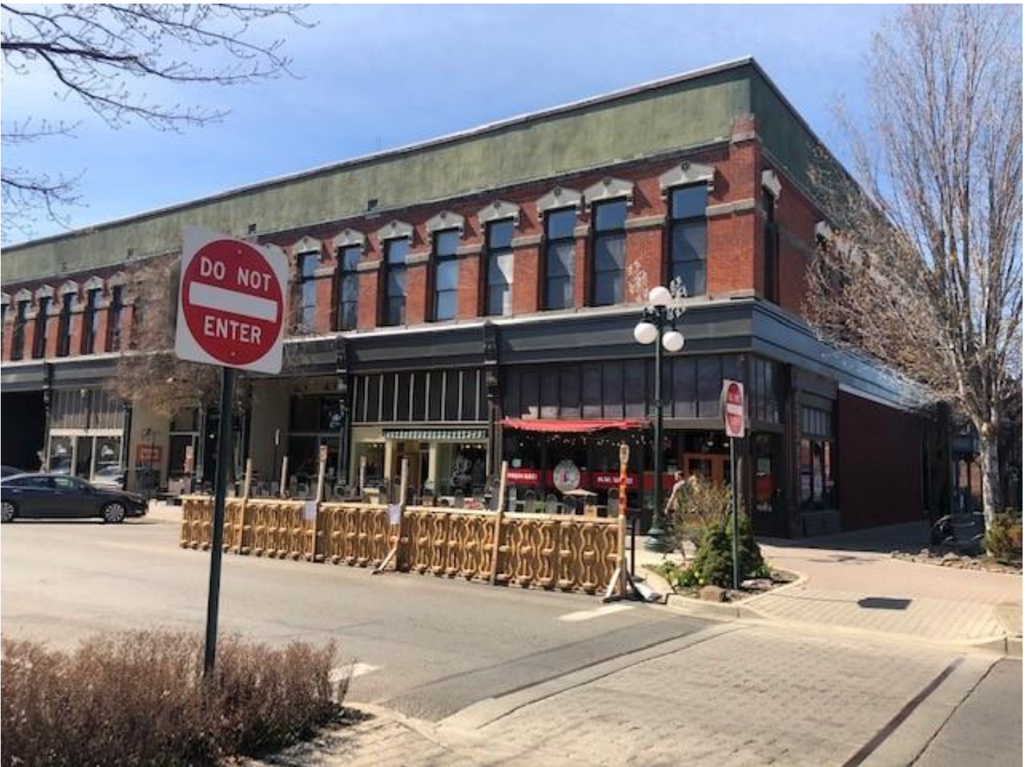
GEDDIS BUILDING – NEAR COMPLETION
