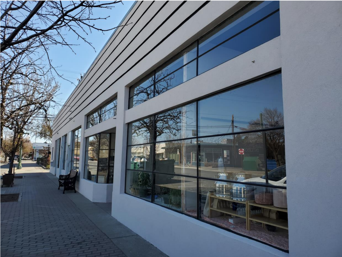
McCORMACK BUILDING WINDOWS AFTER
