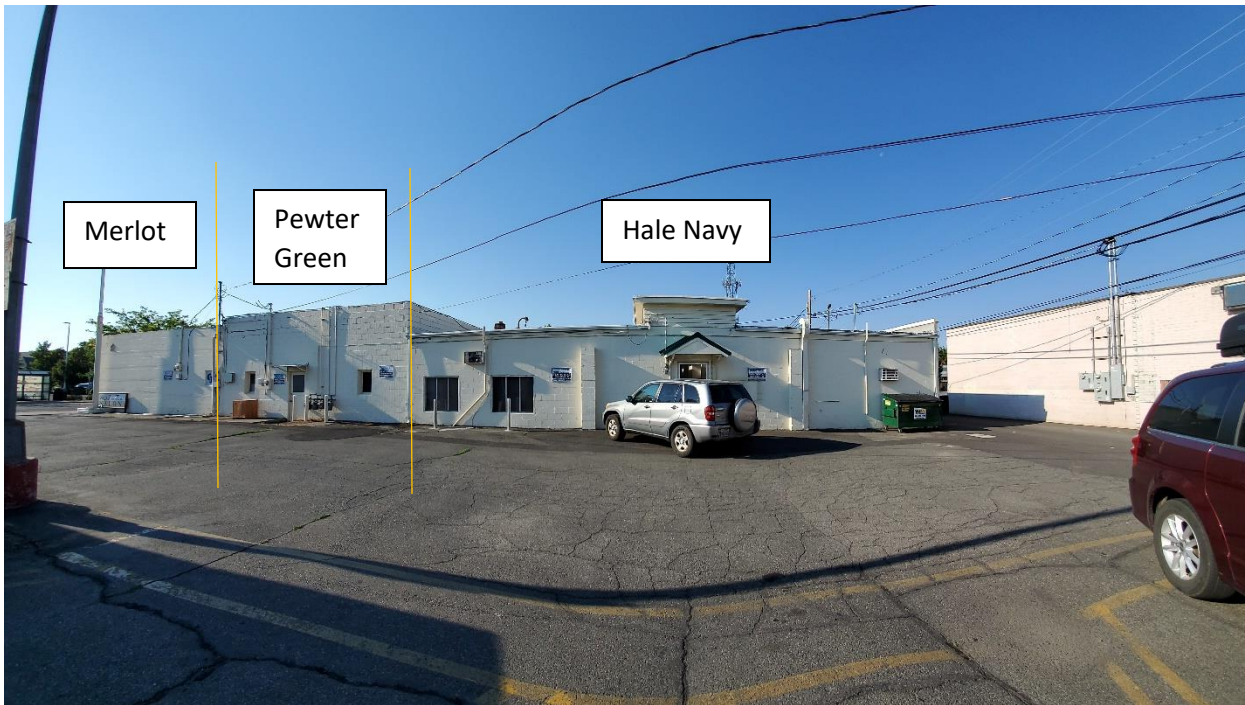
Back of Building- Visible from Ruby Street
