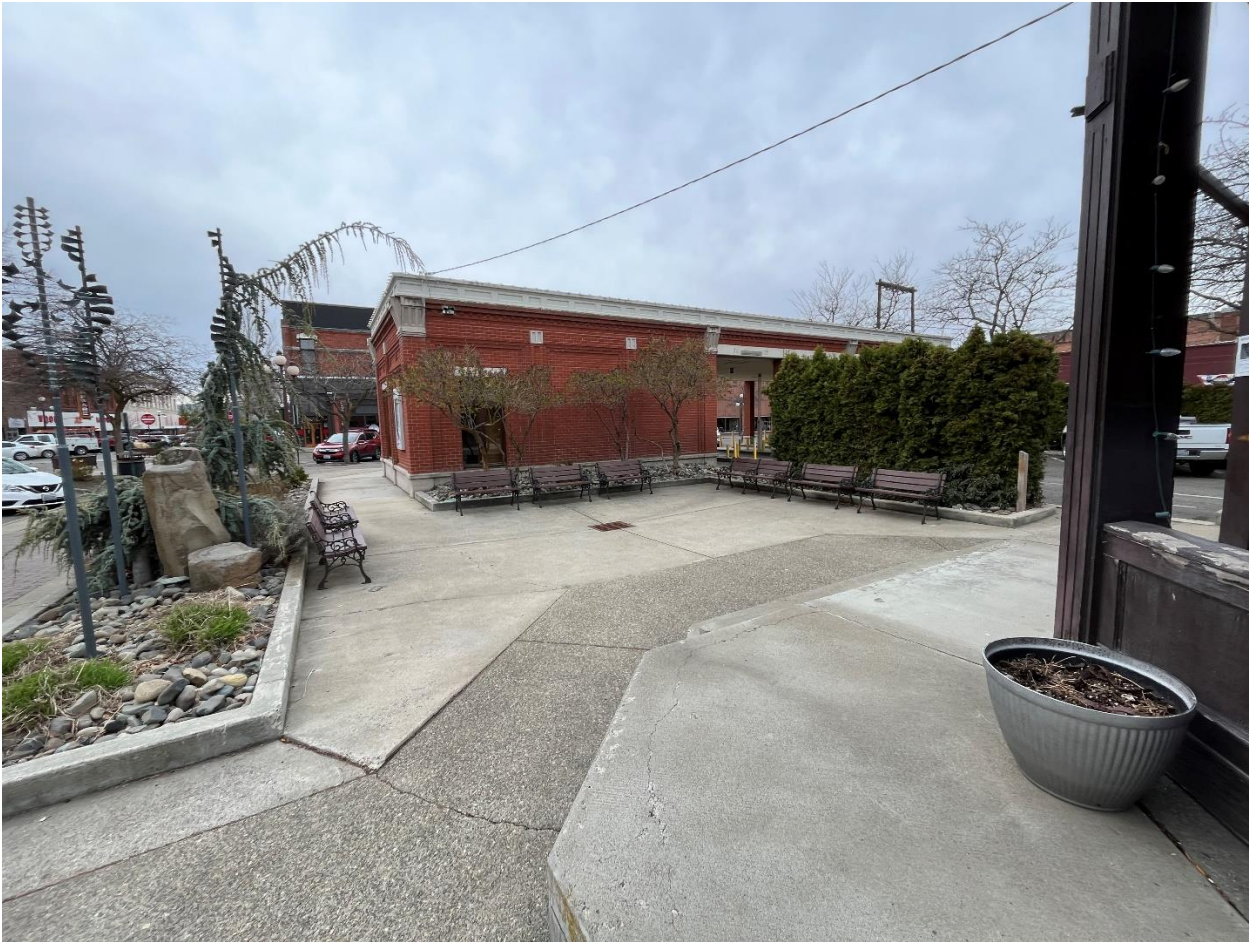
Old Bank Building
