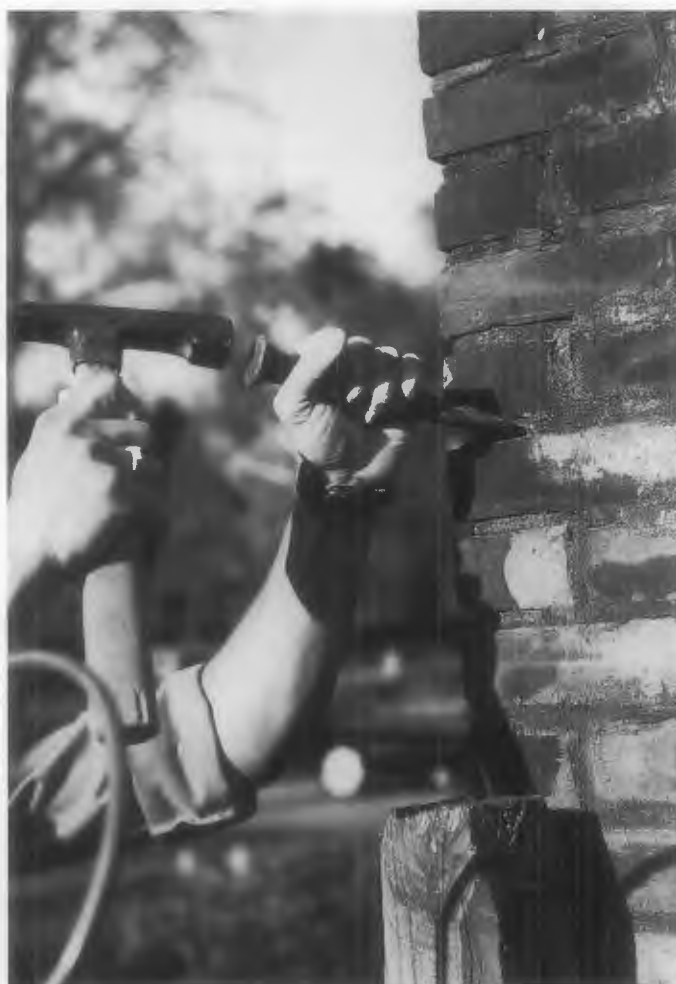
Figure 10. Using a hammer and masonry chisel is the least damaging and, thus, generally the preferred method of removing old mortar in preparation for repointing historic masonry. Photo: John P. Speweik.
