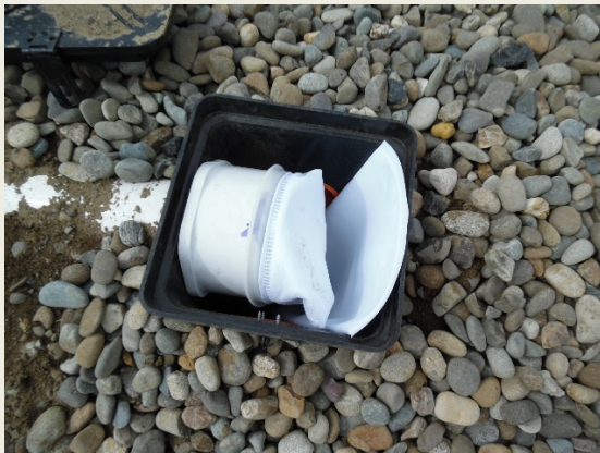
Step 5, install socks in all 8 outfall catchments
