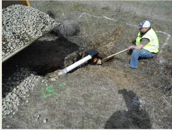
Step 2, make and install outfall equipment
